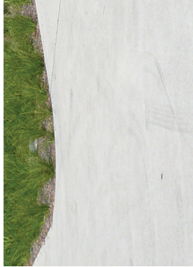
INSITU CONCRETE PATH
